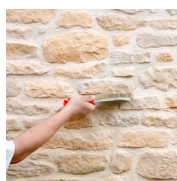
3 - Brush and apply Water repellent
