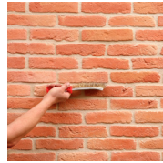
3 - Brush and apply Water repellent
