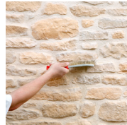
3 - Brush and apply Water repellent
